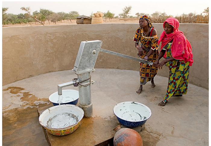
Covered borehole wells help protect water from contamination, making it safe to drink.
