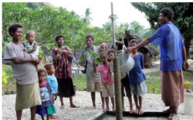
The water tap installed in Delma’s village.
