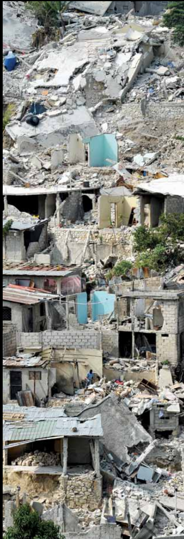
Destruction of homes on the hill side after the 2010 Haiti earthquake. Thousands of people were injured and killed in the falling rubble.
