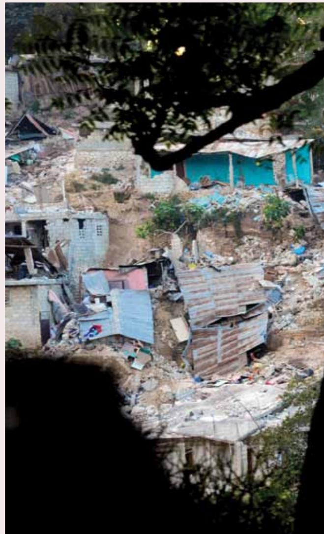
Unsafe, poorly built houses led to the collapse of this whole hillside in Haiti.
