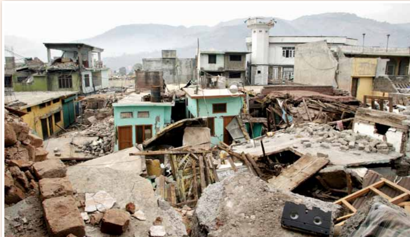
The destruction from the 2005 Pakistan earthquake made it impossible to even walk down the street in this town. Over 70,000 people were killed in this disaster.
