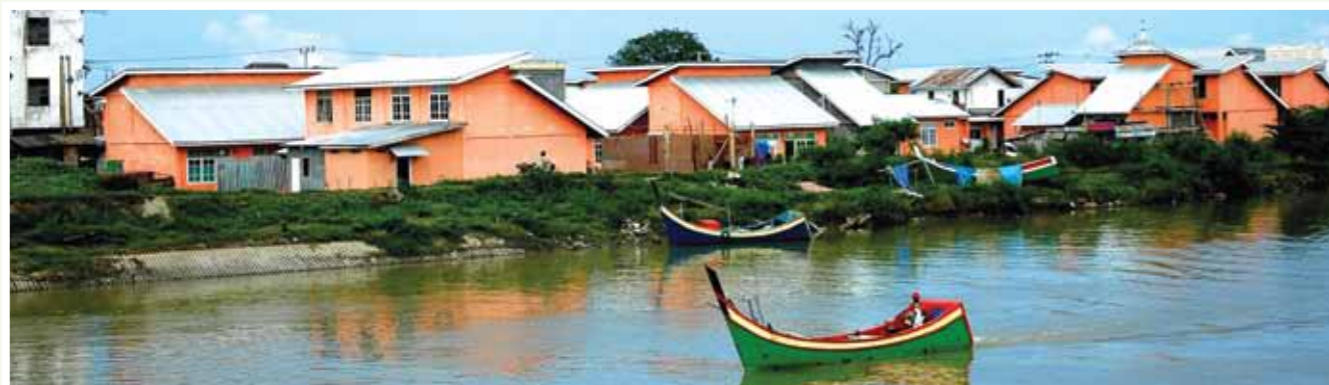
Two years on, this same town had been rebuilt. World Vision has worked with the local community to rebuild houses, schools and roads.
