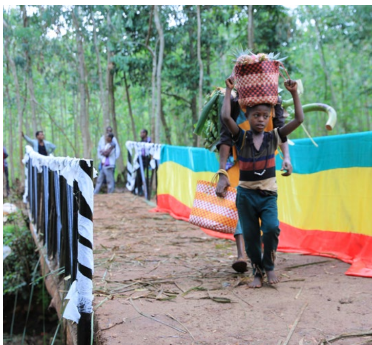
After being destroyed during the conflict, this bridge was reconstructed as part of the connector projects – allowing travel and trade to resume and bringing Gedeo and West Guji communities back together.
