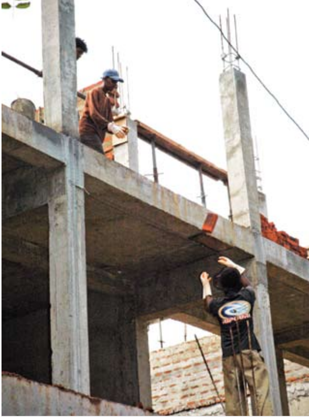
Buildings are reconstructed following the 2004 Indian Ocean tsunami.
