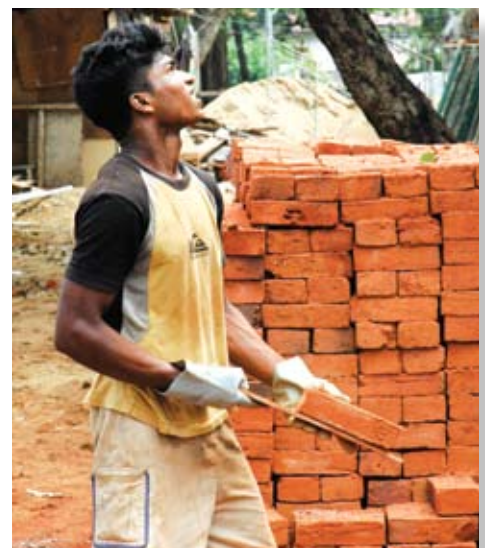
Workers receive skills training to rebuild homes and buildings following the 2004 Indian Ocean tsunami.
