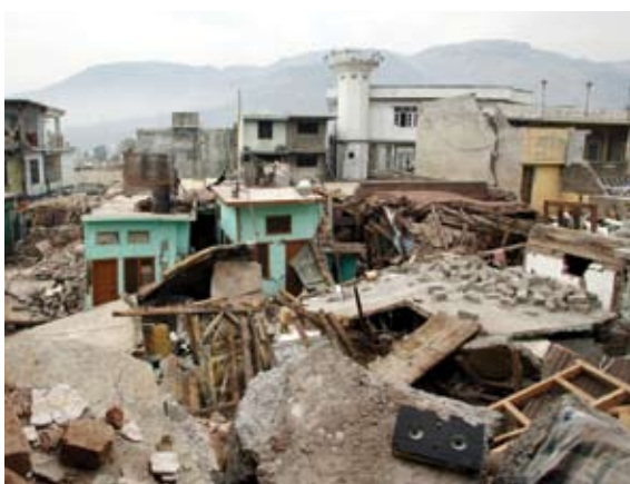
Over 70,000 people were killed in the 2005 Pakistan earthquake. Many people lost their lives due to the collapse of poorly constructed buildings – including schools.
